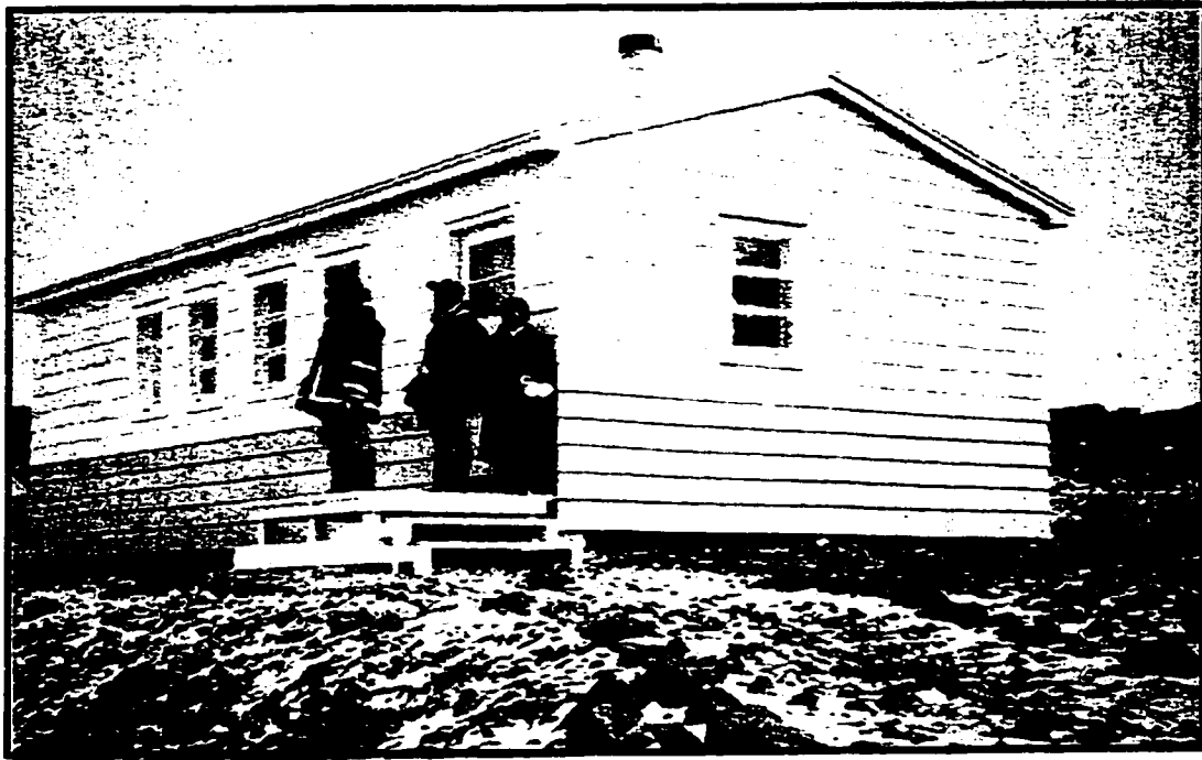
FIGURE 34. Inuit family members stand in front of a new multi-bedroom bungalow in Cape Dorset (after Dept. Of Northern Affairs and National Resources 1960:44)
