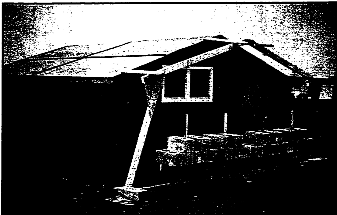
FIGURE 33. Prototype of rigid frame house built by National Research Council of Canada for use by Inuit families (after Dept. Of Northern and National Resources 1960:63)
